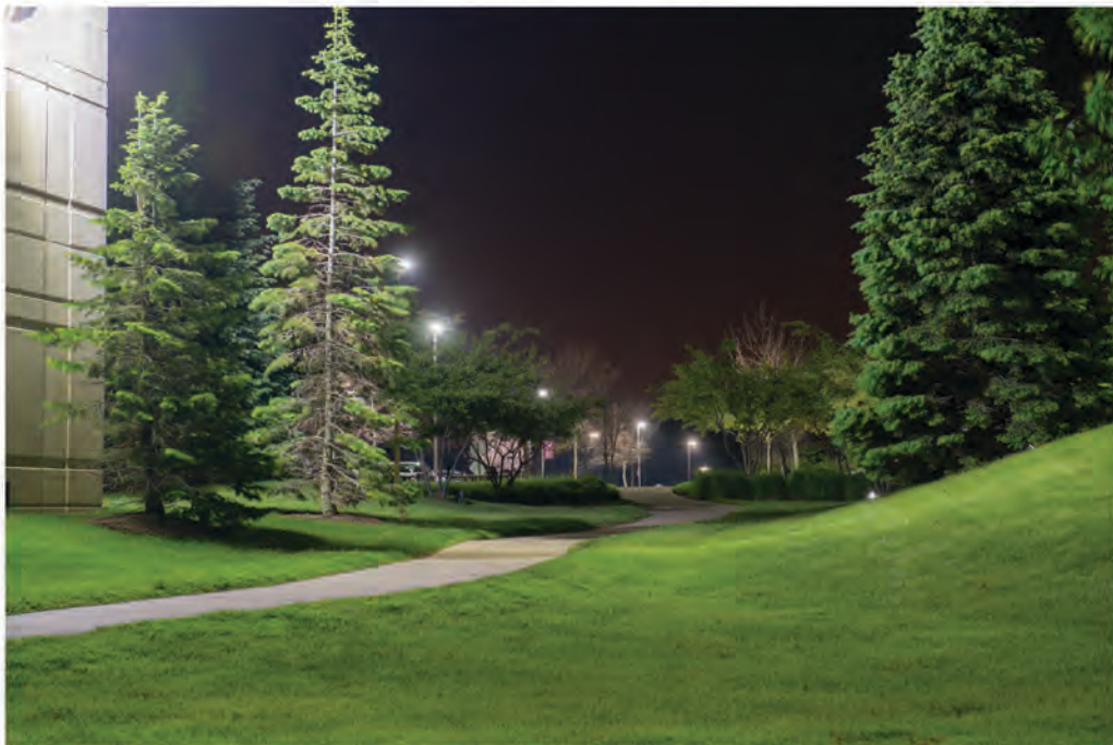
LED luminaires provide uniform light, increasing visibility and improving campus security
